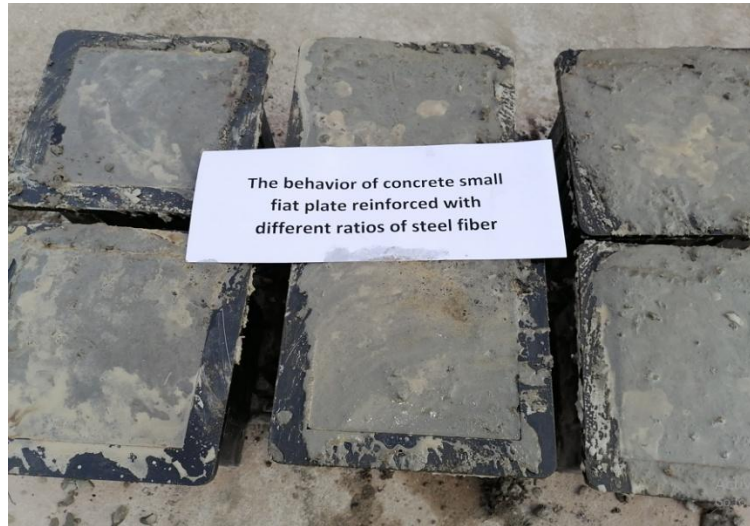
Figure 4. Casting The Mold
