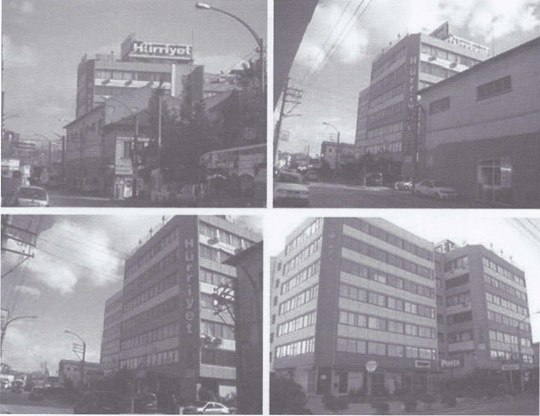
Photo. 3- General view of the İzmir Hürriyet Business Center Building, (Aksoy
