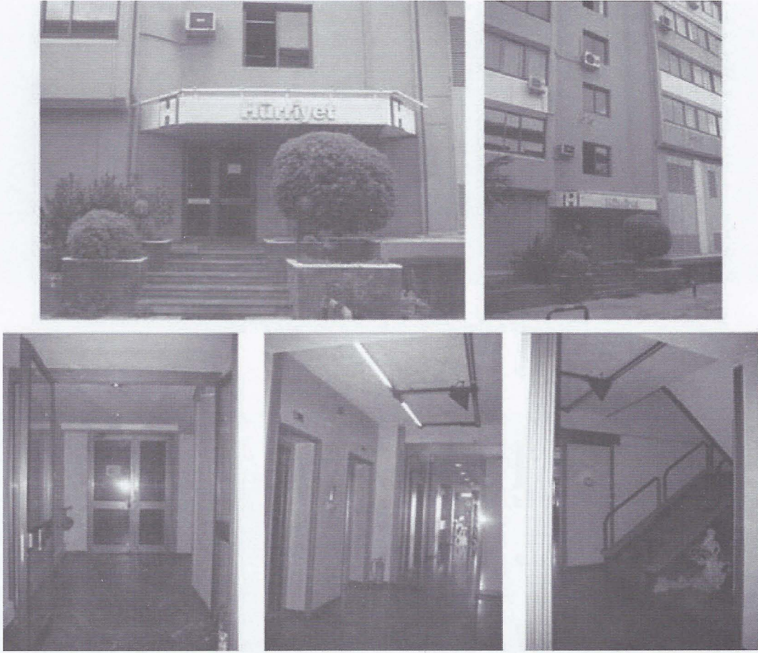
Photo. 5- External view and interior view from service units (Ç.)
