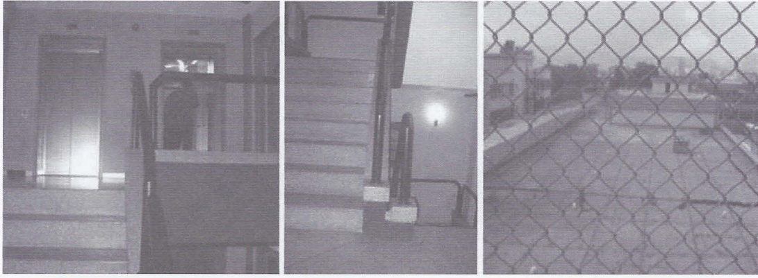
Photo. 7- A.View to vertical circulation areas and b.Terrace roof (Ç.)
