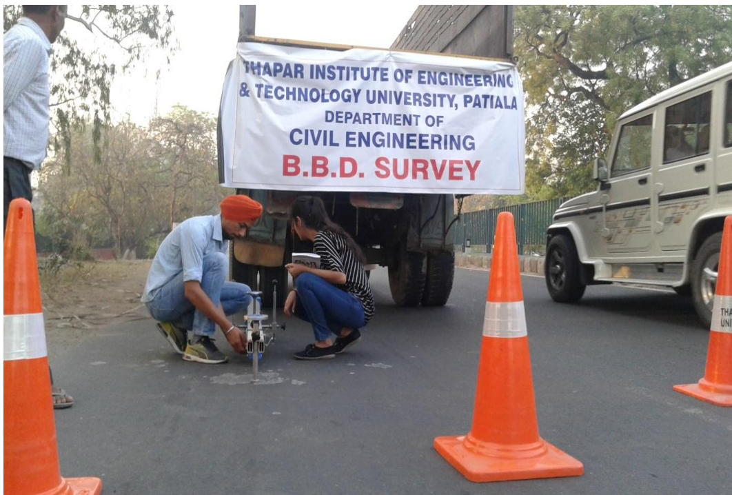
Fig. 2. Benkelman beam deflection test
