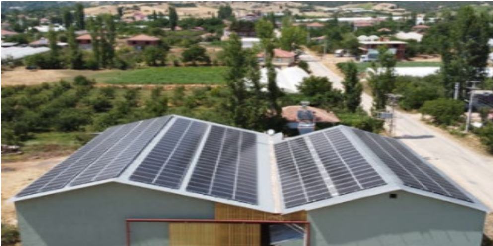
Figure 3. A picture of the power plant being studied.
