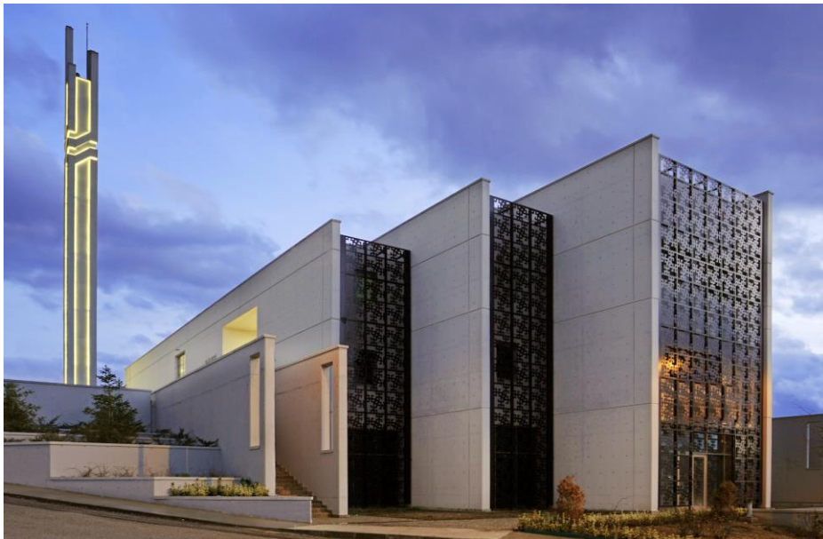
Fig. 12 - Looking at Salih Bezci Mosque Complex from a west-northwest direction.
