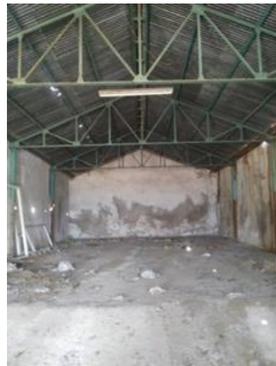
Figure 9. Iron profiles and beams along the long side of the structure
