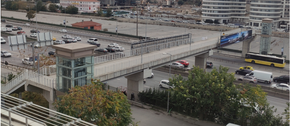
Figure 1 - Studied bridge: Istanbul Medeniyet University pedestrian overpass bridge
