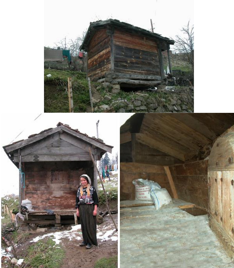
Figure 13, 14, 15. A typical ambar structure Madenler Village – Alaçam / Samsun (photographs belongs to the author).
