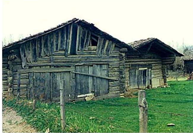
Figure 27. Barns from Kastamonu Region (photo belongs to the author)
