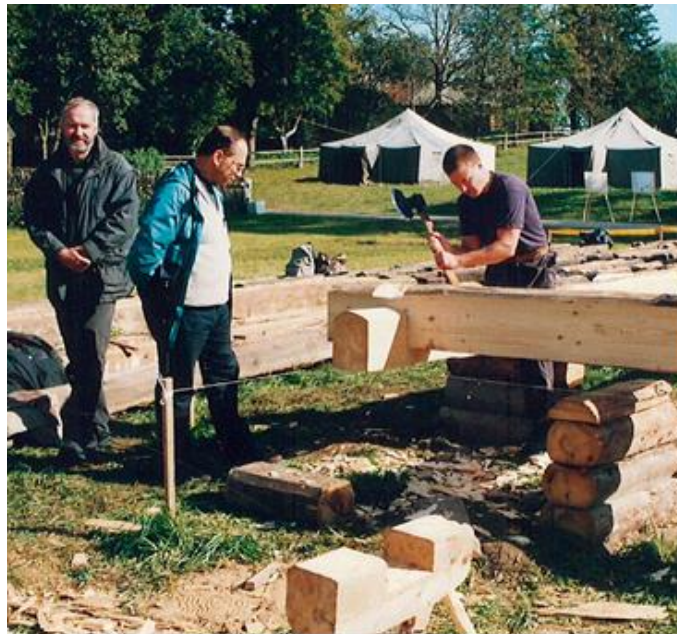
Figure 20. A traditional way of corner binding in Lithuanian log house (photo belongs to the author / 2001).
