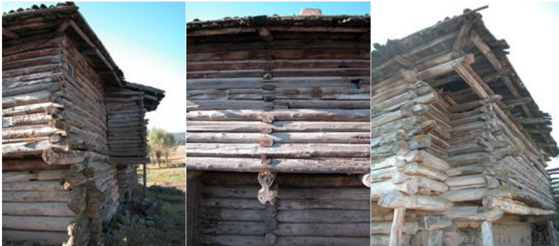
Figure 7, 8, 9. Details from joining connections of different log buildings located high plateaus of Anatolia. (photographs belongs to the author).
