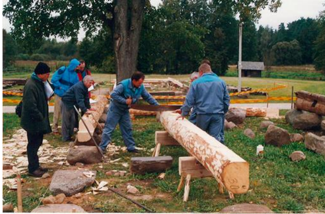
Figure 21. A traditional way of preparation of timber log before construction in Lithuania (photo belongs to the author / 2001).
