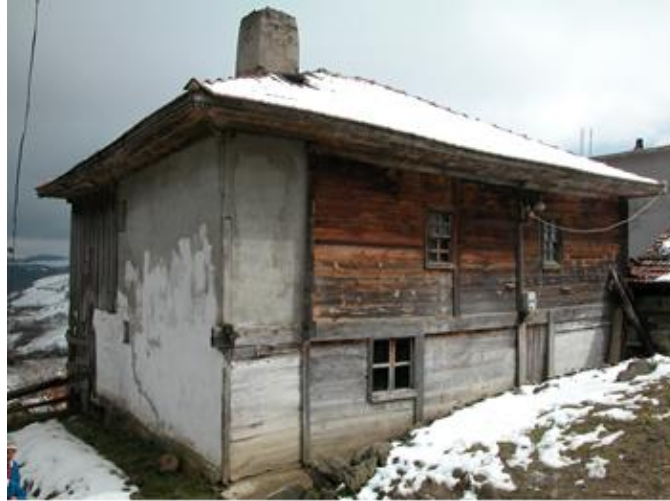
Figure 4. A typical two storey house from Alaçam mountain village (photo belongs to the author).
