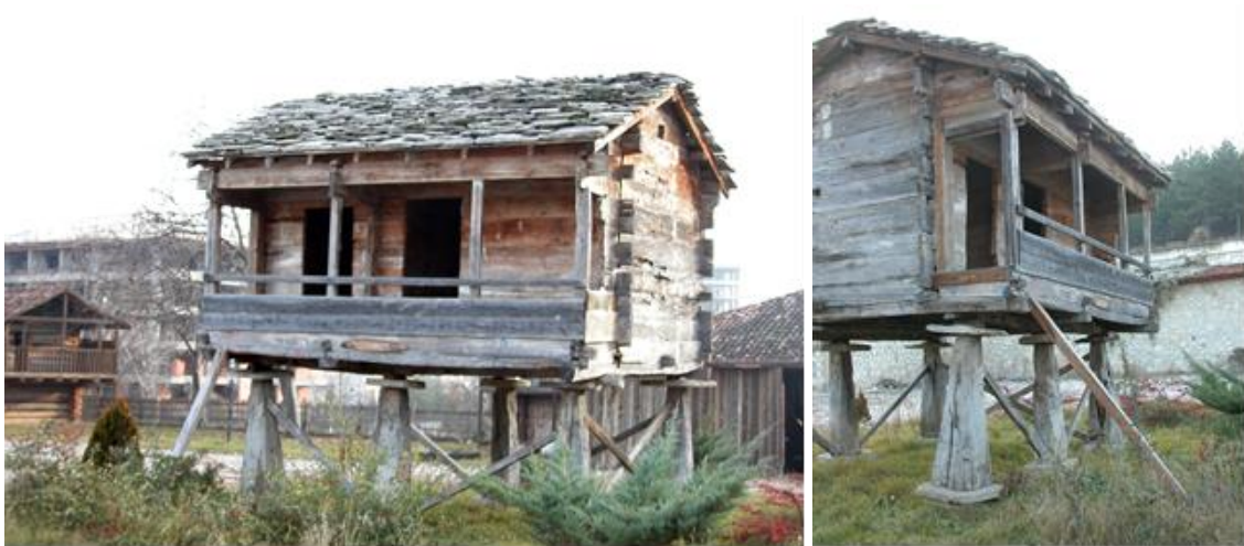
Figure 17, 18. A typical serender structure Kastamonu (photos belongs to the author).
