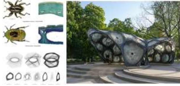
Şekil 3. ICD/ITKE Research Pavillion 2013-2014 (Figure 3. ICD/ITKE Research Pavillion 2013-2014)
