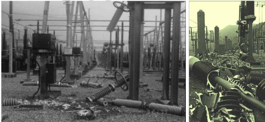
*Figure 1 - Partial collapse in power stations during the 1999 Chi-Chi Taiwan earthquake [2]*
