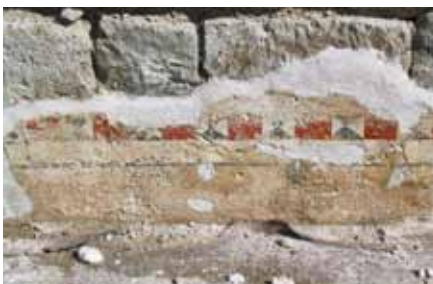
Figure 22 Partially preserved wall paintings in the west edge of the north wall
