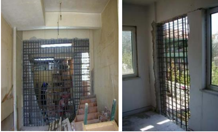
Figure 6. Reinforcement of reinforced concrete frames with cast-in-place curtain walls
