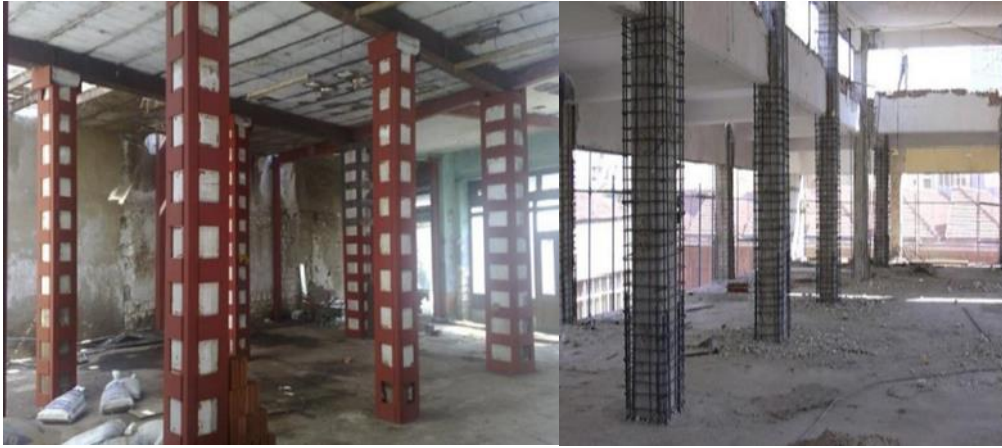
Figure 2. Reinforcement of Columns
