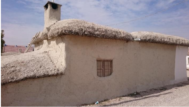
Figure 1. The house constructed with bog bulrush.
