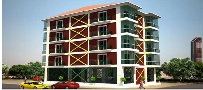
Figure 1. Externally Strengthening of RC Building
