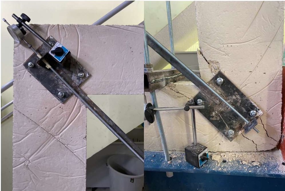
Figure 4. Fixing Steel Lama and Placement of Comparator on RC Frame using Anchor Bolts
