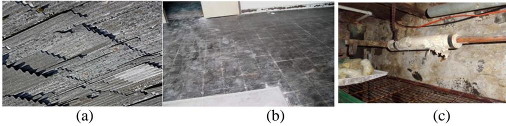
**Figure 4.** (a) Asbestos roofing, (b) Asbestos floor covering, (c) Asbestos pipe (Şahin ve Bingöl, 2022; Tezcan, 2007, T.C. Ministry of Labor and Social Security, 2023)
