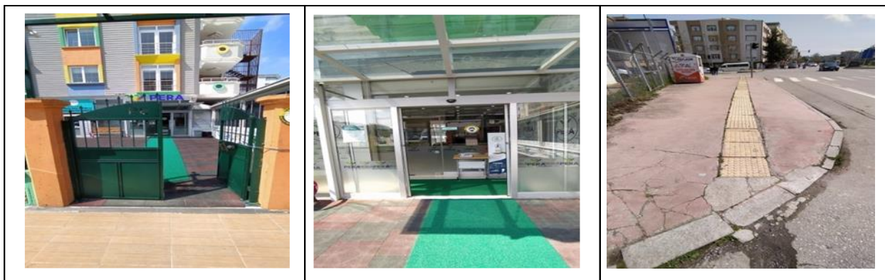
d) Main entrance door
