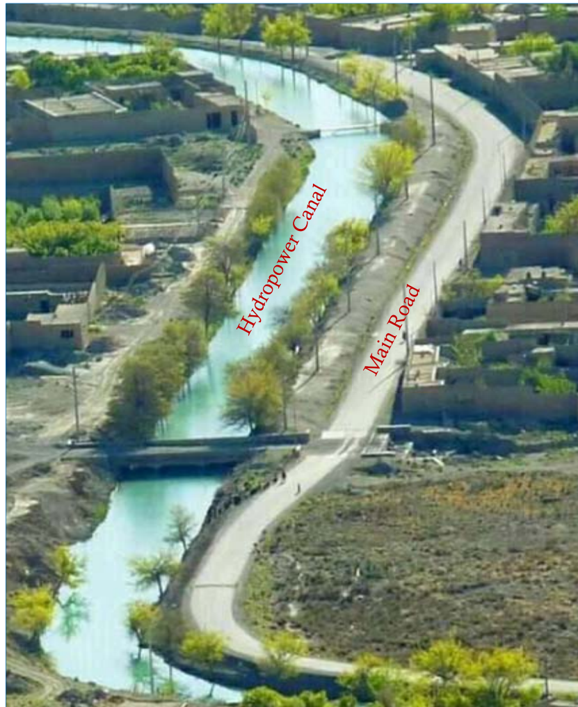
Fig. 7. Chack Hydropower canal
