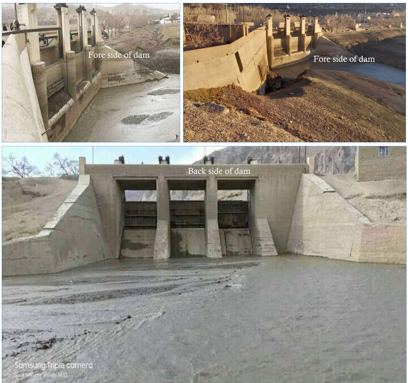
Fig. 6. Different parts of Chack Dam construction
