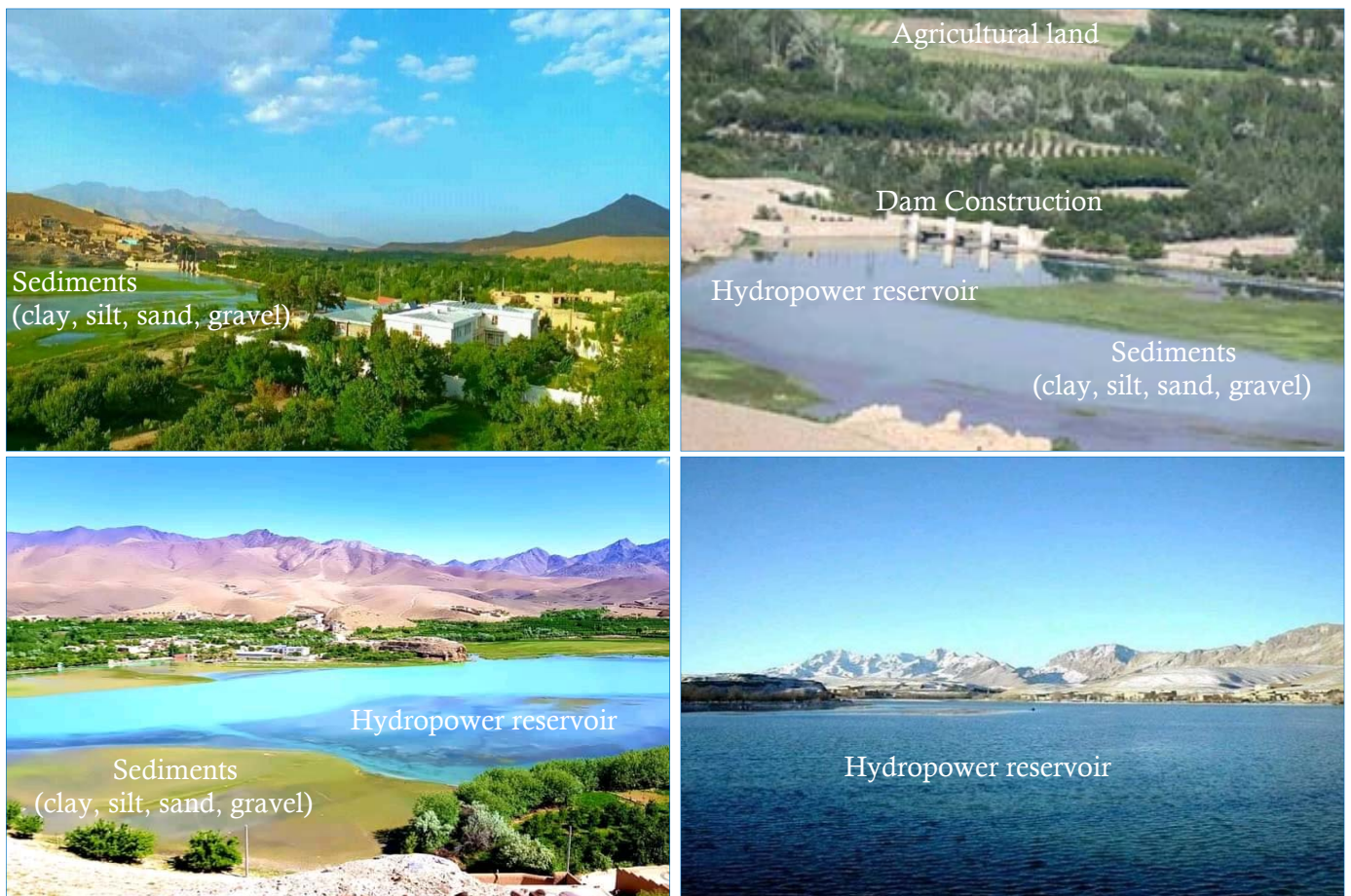
Fig. 5. Different parts of Chack reservoir at the various seasons of year
