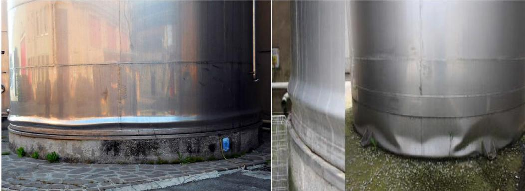
**Figure 7.** Elephant’s foot buckling, Emilia earthquake, Italy, 20 and 29 May 2012 [13]
