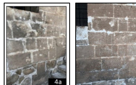
Figure 7. Anthropogenic degradation of Hatuniye Madrasah (Biçen Çelik, 2019)
