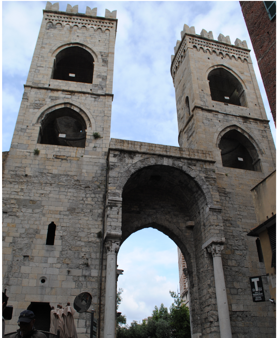
Figure 13: Genoa, city walls, Porta Soprana, pointed arches in the gate and the towers. Photograph: Selin Sur, 2013.
