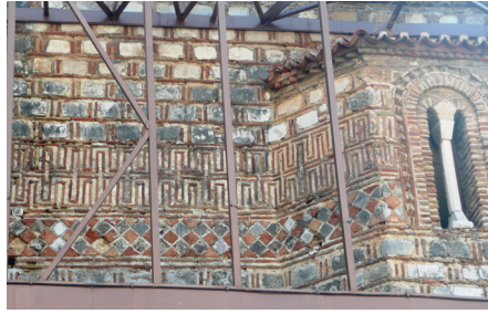
Figure 5: Latmos, İkiz Ada, Katholikon (thirteenth century), wall technique with cloisonné and “brick-filled mortar joints” (left). Photograph: Ufuk Serin, 2003. Arta (Greece), Church of Panagia Parigoritissa (thirteenth century), displaying rich varieties of the cloisonné and champlévé techniques in masonry (right). Photograph: Ufuk Serin, 2010.
