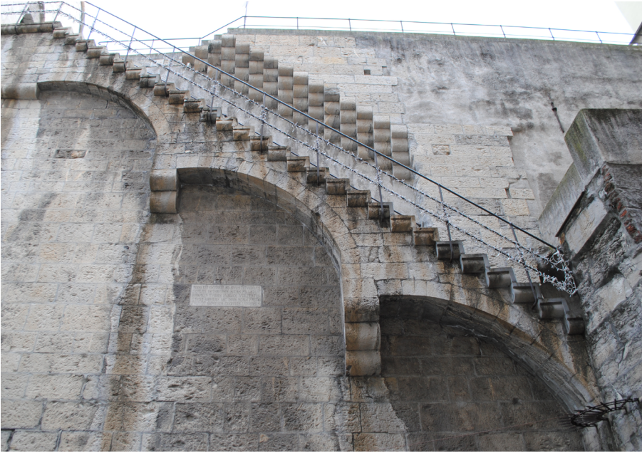
Figure 6: Genoa (Italy), city walls; regular stone masonry of the walls near Porta Soprana. Photograph: Selin Sur, 2013.
