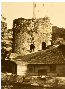
Figure 8: Galata Walls, arches composed of stone and brick in a demolished tower. Photograph: Pascal Sébah, ca. 1870. Suna and İnan Kırcaç Foundation Photography Collection, İAE, FKA_003035.
