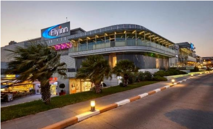
Figure 2. Flyinn Shopping Center Front Facade View [14].
