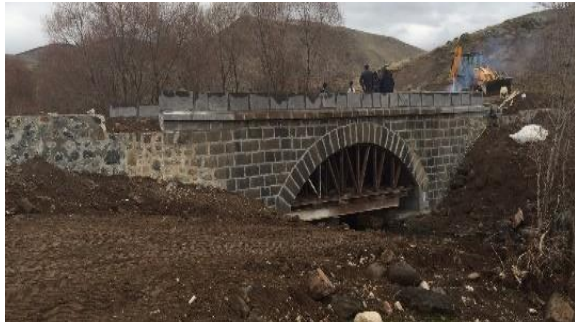
Figure 2. Sultan Hamit I Bridge
