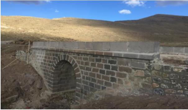
Figure 6. Sultan Hamit III Bridge
