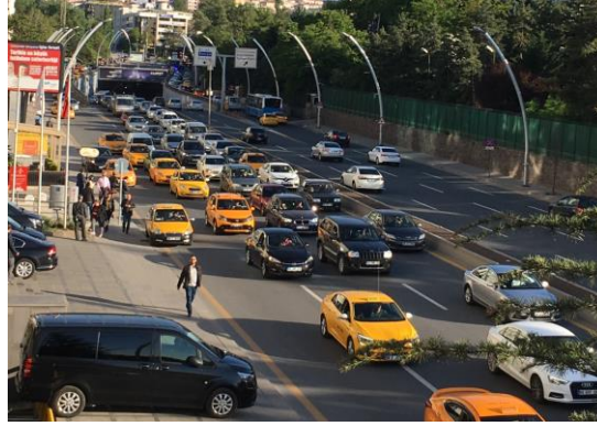
Figure 2. Kuşulu grade separated junction blocking pedestrian crossing at the city center
