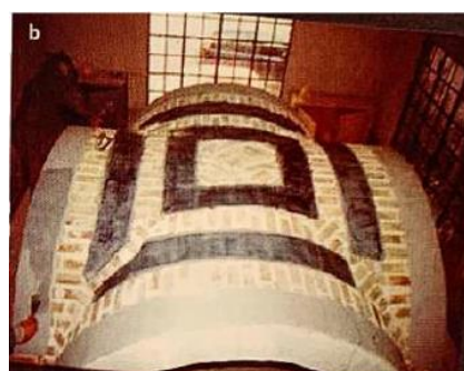
Figure 4. Application of FRP materials (Zakar & Eyüpgiller, 2020)
