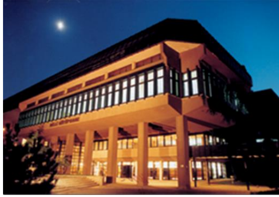
Figure 1. The current building of the National Library [19]
