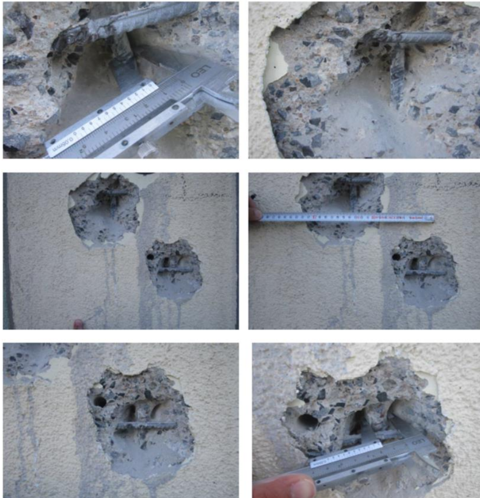
Figure 5. Reinforcement detection by stripping
