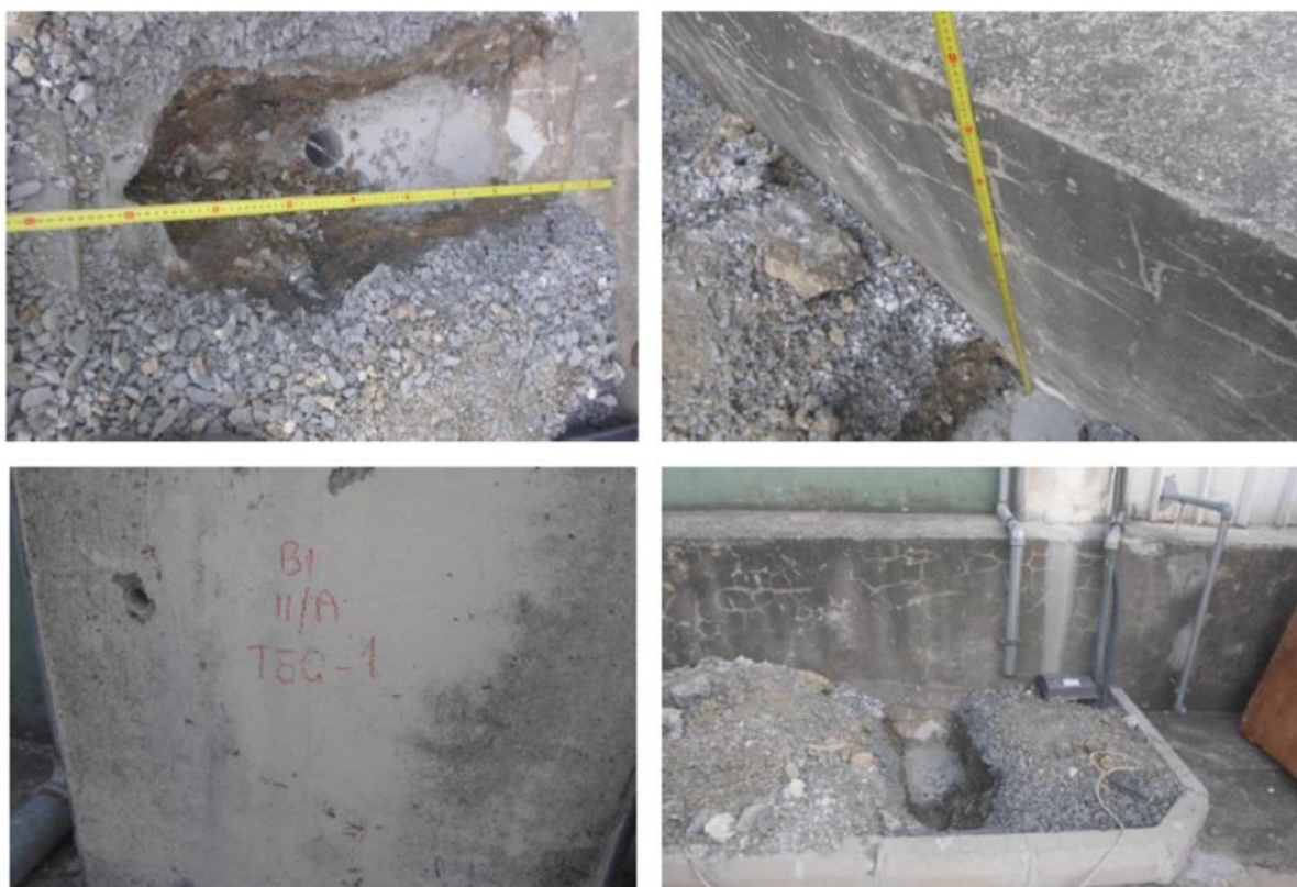
Figure 3. Foundation test pit excavation
