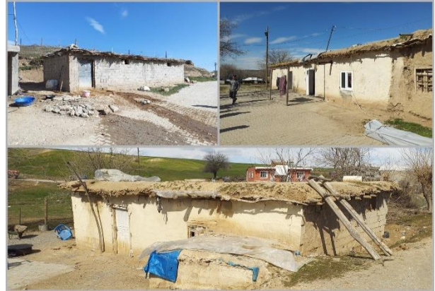
Figure 15. Example of heavy earthen roof with no damage
