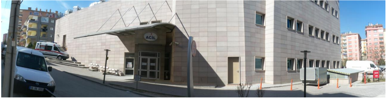
Figure 7. Entrance point of emergency department of Lokman Hekim Hospital
