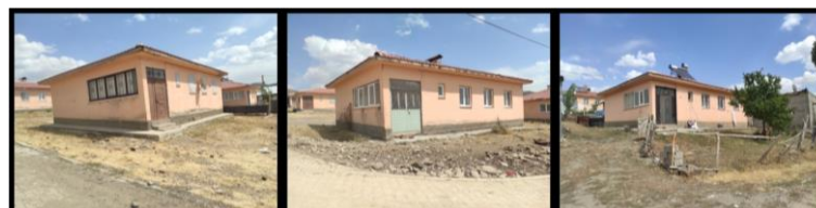
Figure 12. Examples of AFAD houses with enclosed terraces
