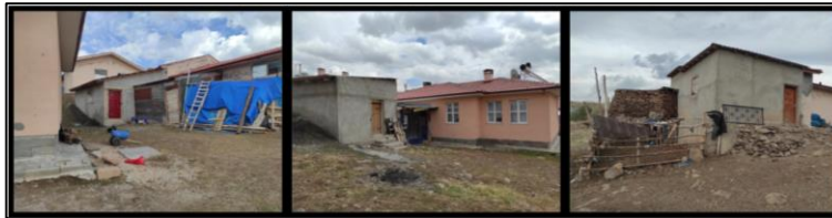
Figure 15. Examples of additional structures such as woodshed/coal storage, garage, tandoor house, etc. added to resettlement houses
