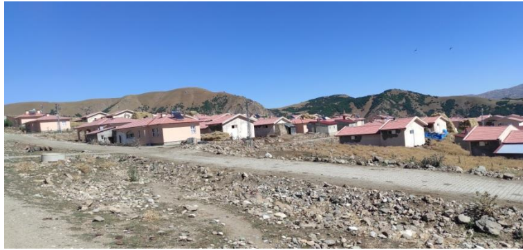
Figure 8. Settlement area of Kalecik village housing units (Photo Archive by T. İnanç)
