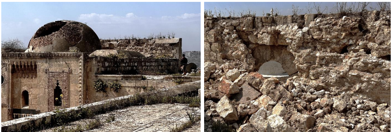
Figure 33. The Partial Destruction of the Dome and the External Façade Wall (Dayoub, 2023©) © Museum for Islamic Art in Berlin
