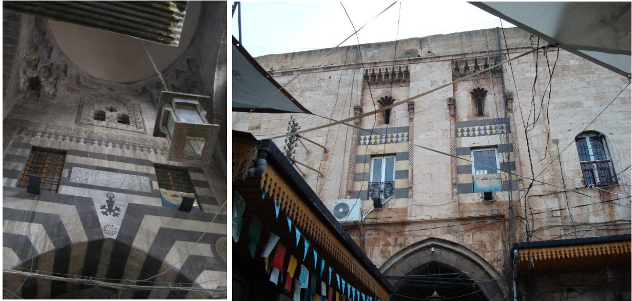
Figure 27. The External Façade, to the left, and the Courtyard Façade, to the right, of Khan al-Gumruk's Entrance (Kasmo, 2011)
