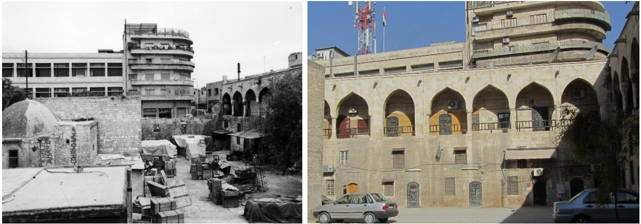
Figure 30. The Eastern Section of the Northern Wing after its demolition (David, 1982©) and after its reconstruction (Kasmo, 2010) © Museum for Islamic Art in Berlin
