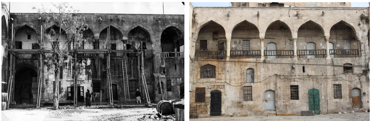
Figure 29. The Northern Section of the Eastern Upper Portico during the 1939 Repairs (Michel Ecochard Archive ©) and after (Kasmo, 2010)
