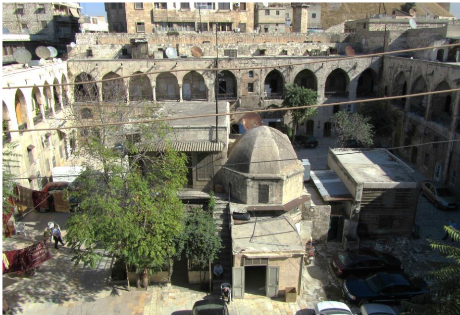
Figure 9. A General View of the Khan's Courtyard from West (Kasmo, 2010)
