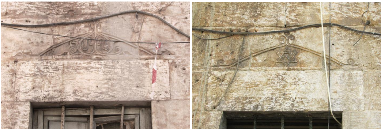
Figure 28. Carved Ornament above the Openings overlooking the Courtyard (Kasmo, 2010)
