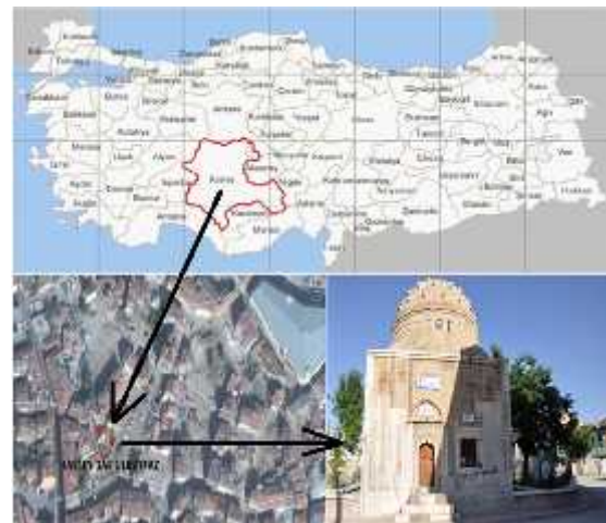
Figure 1. Location and general appearance of Hasbey Dar'ülhuffaz
