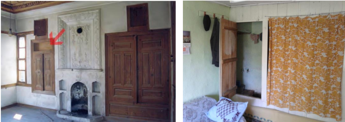
Figure 9. Gusülhane with its doors closed in a Çorum House (left) [20], Gusülhane with its door open in a Yalvaç house that still in use today (right) [49]
