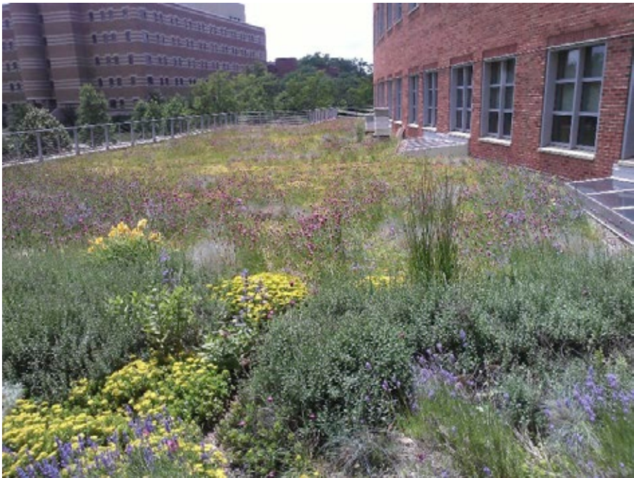
Image: Green roof on Penn State University (self-credit)
