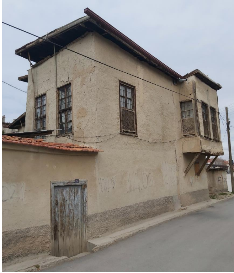
Figure 30. 19 th Century traditional konya house (Location: Island: 522, Plot: 16 (KKBS,2023)).
