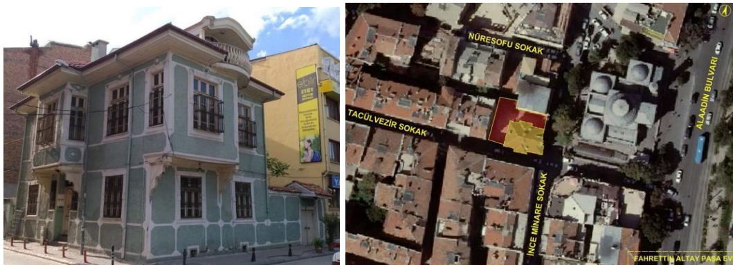
Figure 22. Fahrettin Altay Paşa house and location (Island: 452, Plot:28 (KKBS,2023)).
