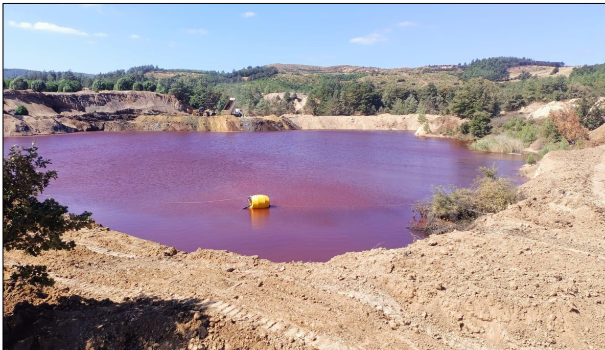
Figure 1. Abandoned coal mine site in çanakkale çan region with amd formation observed. turning to red color after oxidation with atmospheric weather conditions.
