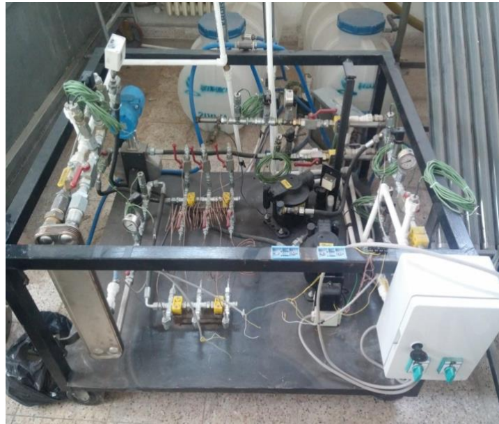
Figure 2. Heat pump system to be tested
