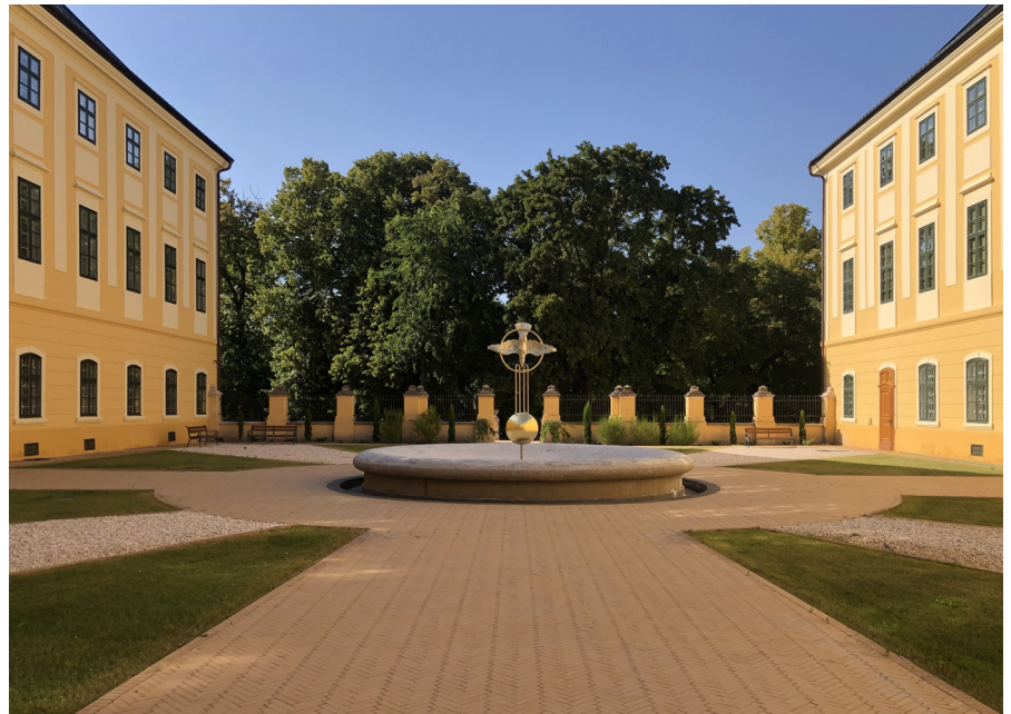
Figure 2 The inner courtyard of the Archbishop's Castle in Kalocsa with the fountain. Work in progress. Photo by Márta Vörös.
