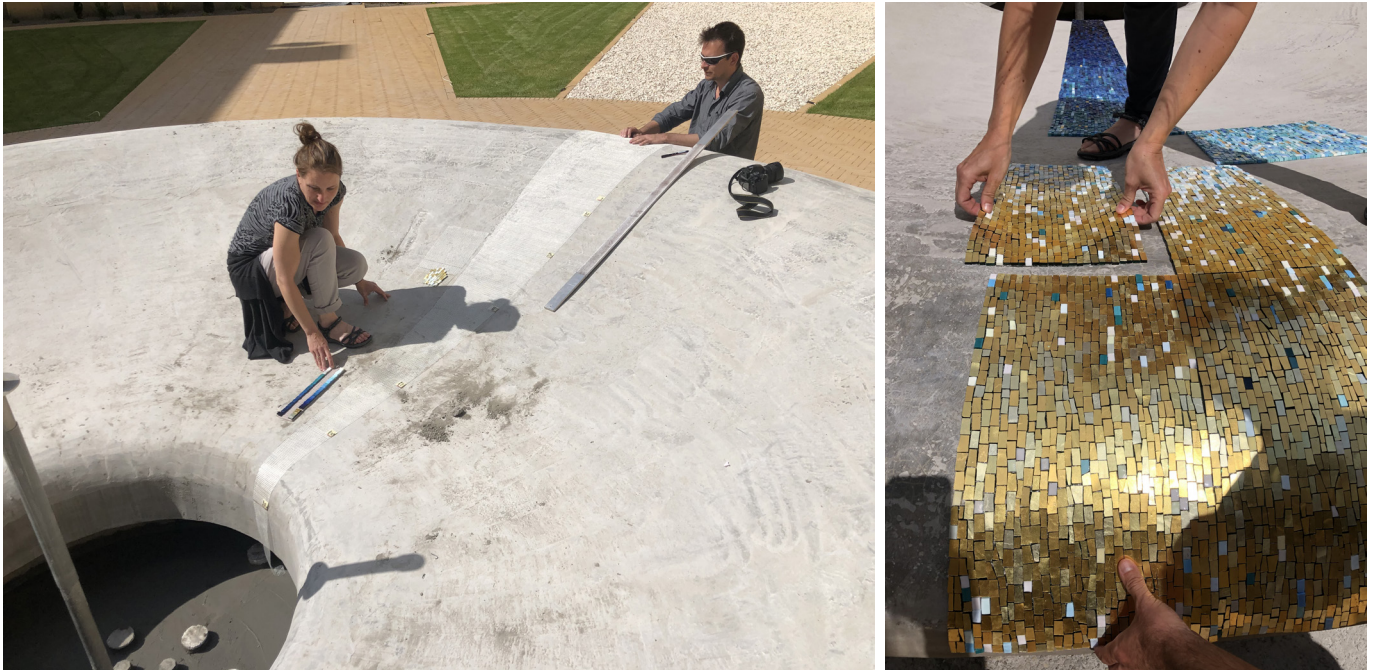
Figures 9a-b On-site measuring process for planning the best fitting size of the elements and trial to the arrangement of the firstly made sections following the measurements. Photos by Márta Vörös.
