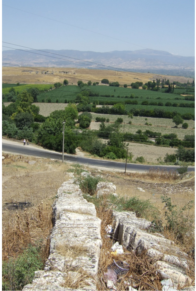
Fig. 5. Travertine blocks of siphon system to Terminal 1, courtesy of the author.
