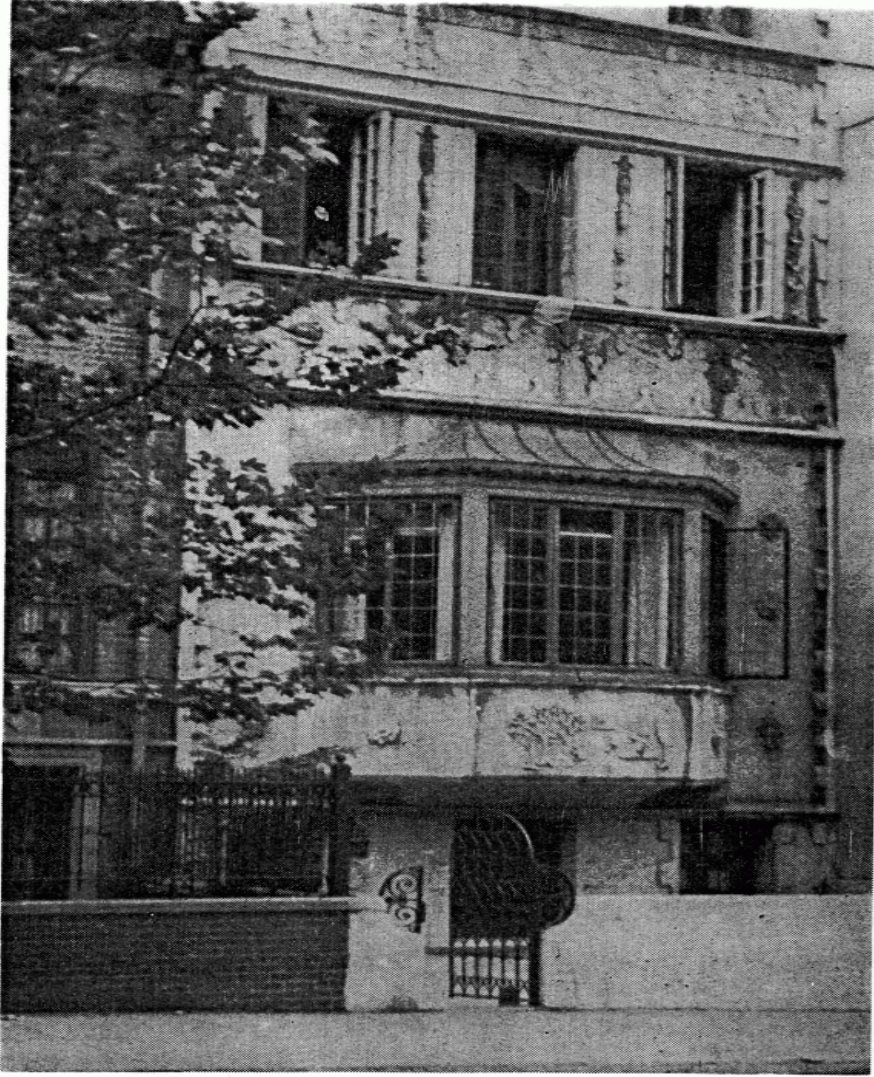
Residence of Mr. and Mrs. L. S. Chanler now Caravan House
