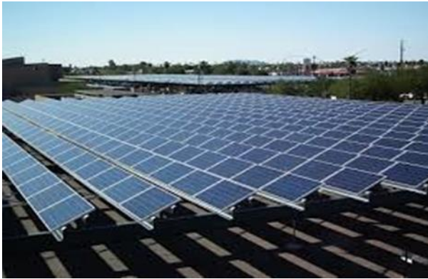
Figure 13. Integration of framed PV systems on flat roofs [23].
