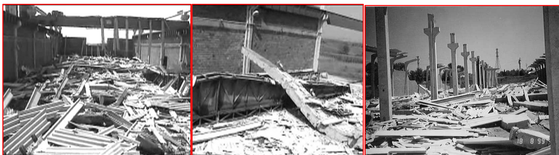
Figure 12. Prefabricated Structural Element Factory
