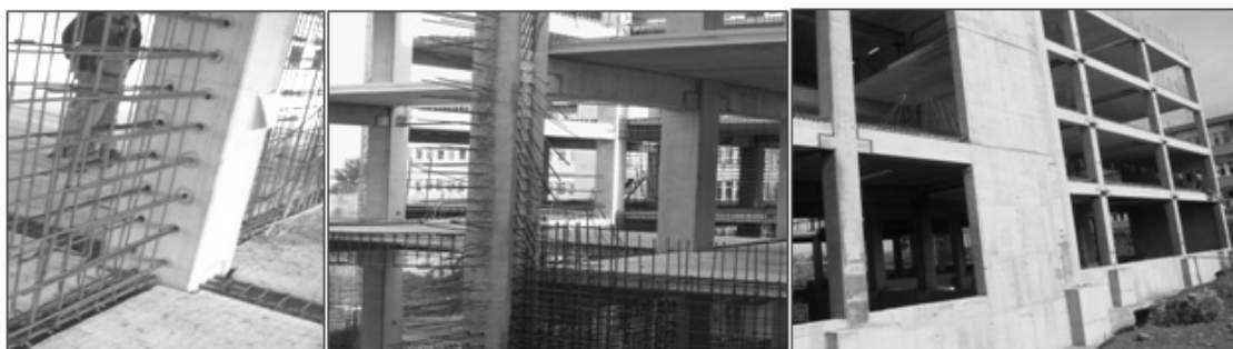
Figure 11. Photographs of RC Wall construction on a prefabricated structure
