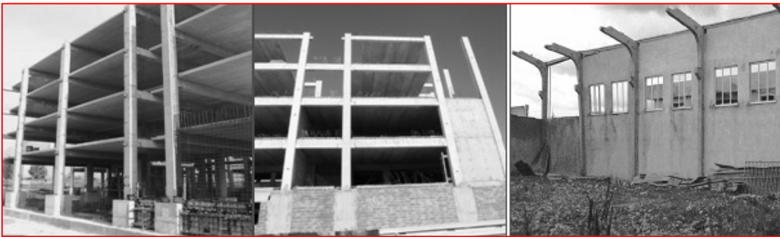
Figure 4. Photographs of multi-story precast building Facilities
