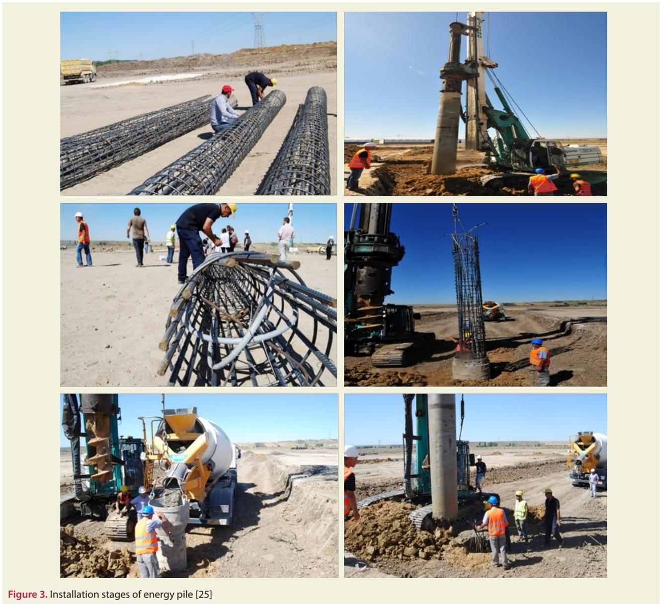
Figure 3. Installation stages of energy pile [25]
