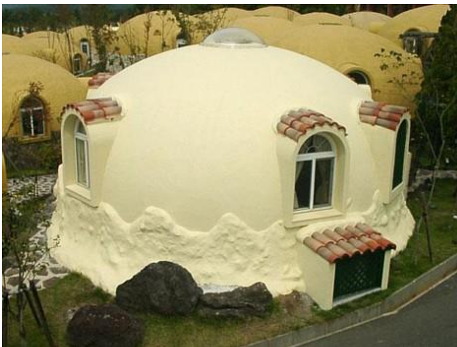
Figure 13. View of a Prefab Styrofoam Dome House; There are More Units Behind the Dome House (Trendir, 2016).
