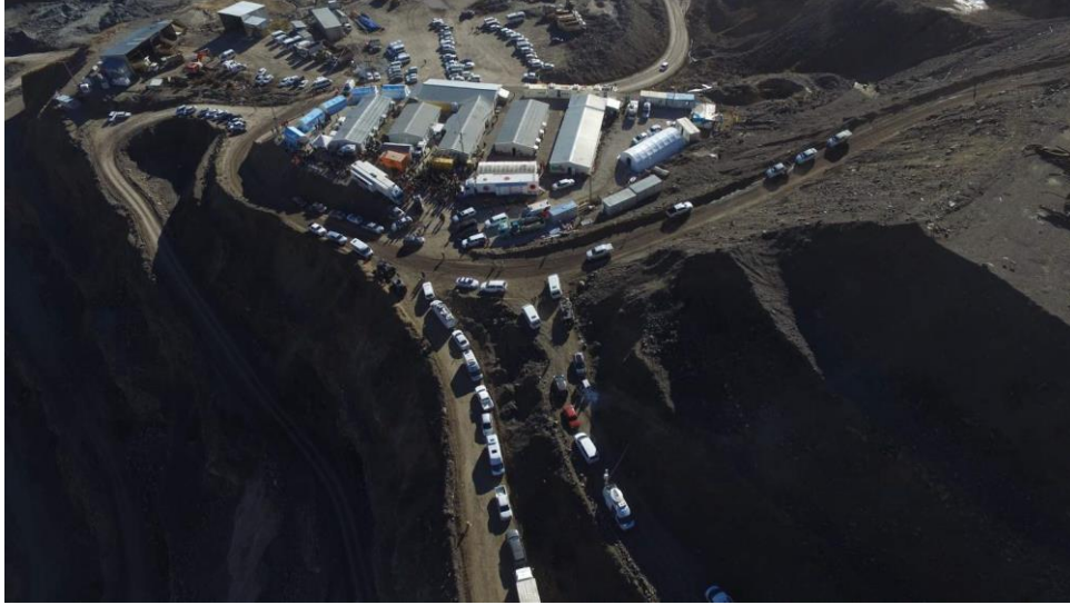
Figure 3: Landslide Area of Mine Field
