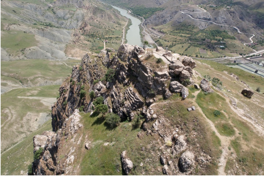
Figure 8: Foundations of the terrace walls in the northern sector of the Upper Citadel.
