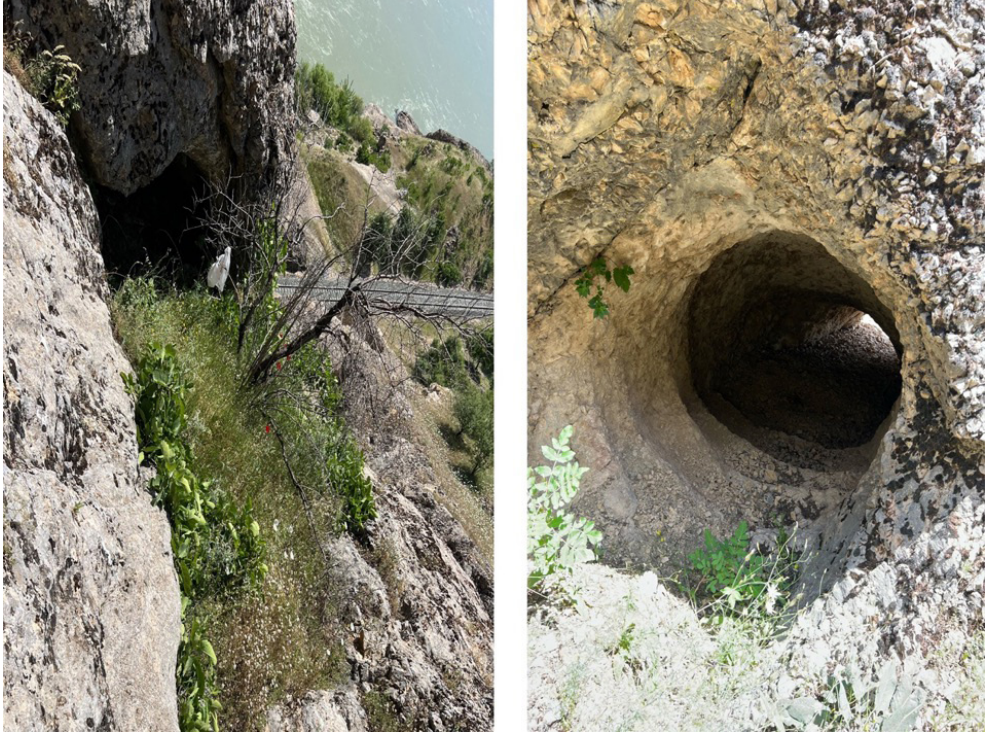
Figure 23: Entrance to Stepped Rock-cut Tunnel C (left), view from inside the tunnel (right).
