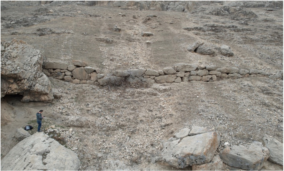
Figure 11: Lower Citadel fortifications, view from the east.
