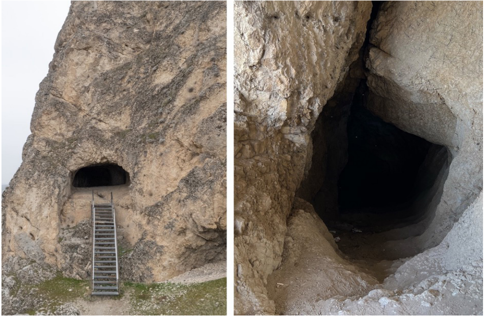
Figure 21: Entrance to the gallery leading to Stepped Rock-cut Tunnel A (left), entrance to Tunnel A (right).
