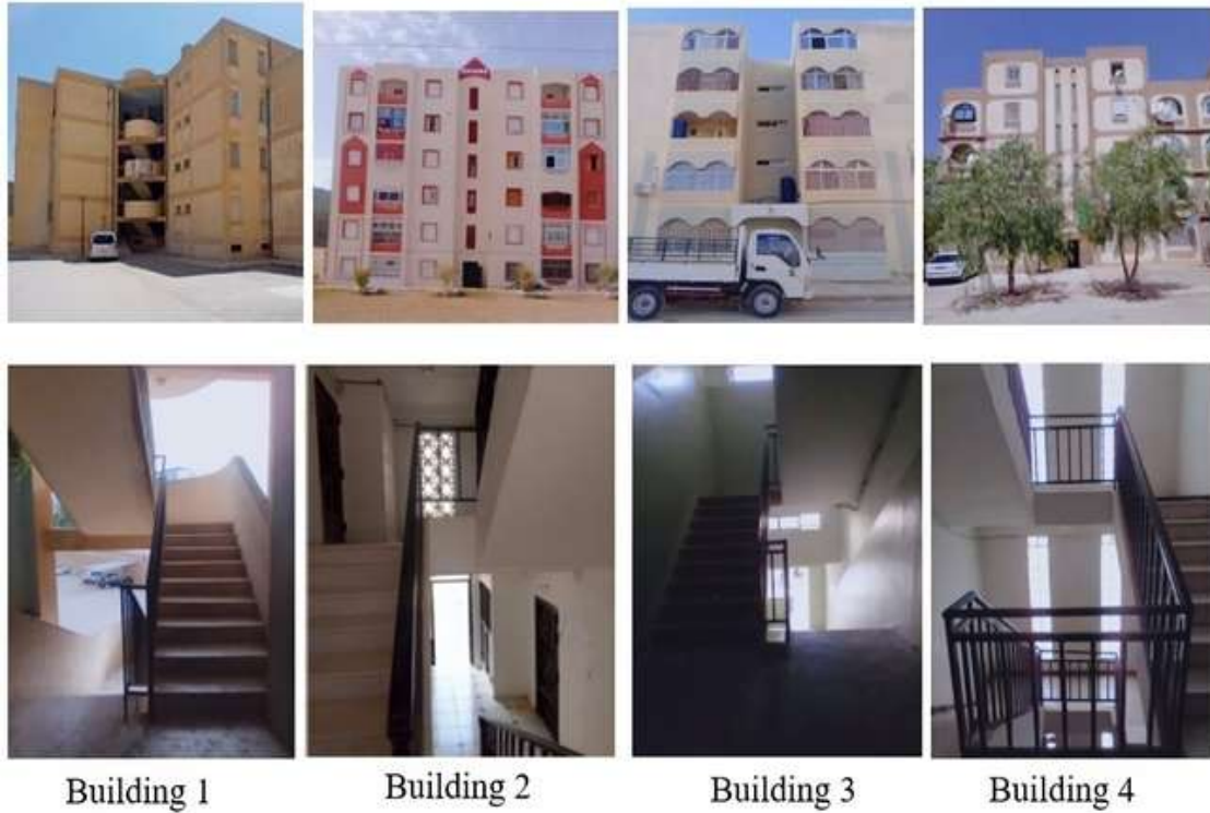
Figure 2. Surveyed Buildings. Source: Author
