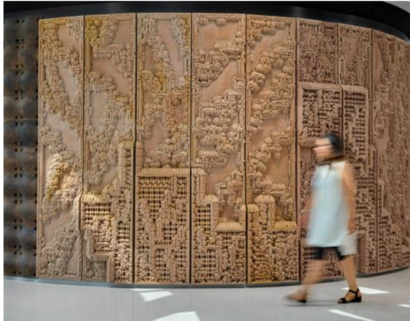
Figure 3. 3D-printed Wall, Wark, B., Photo Credits: Wark, B., [11].
