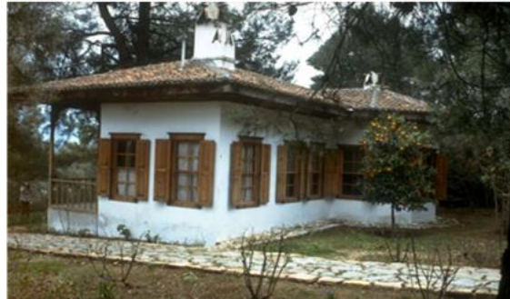
Figure 6. Side elevation showing the wooden eaves; Mugla chimney and rectangular wooden Windows (Çakırhan, 2005).
