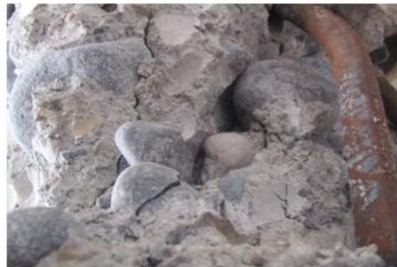
**Fig.25.** Examples of poor concrete quality
