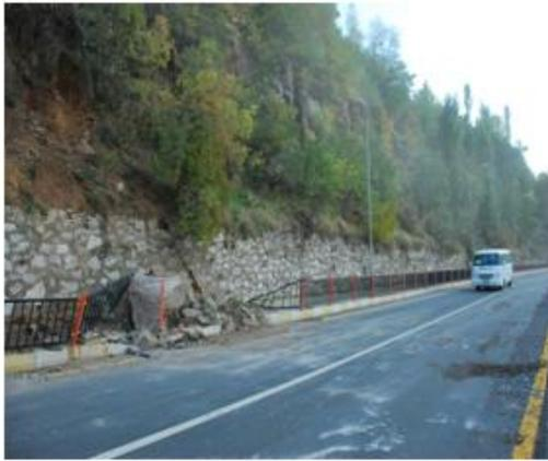
**Fig.11.** Rockfall damage
