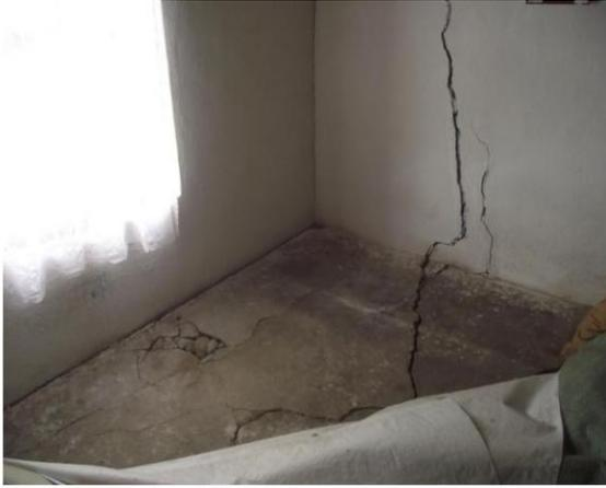
**Fig.23.** Floor and wall damage in ground story
