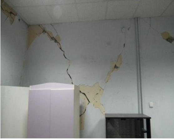
**Fig.15.** Typical structural wall damage
