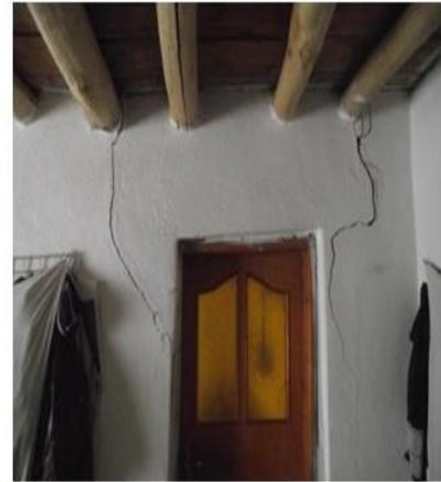
**Fig. 22.** Wall damages in masonry and RC buildings
