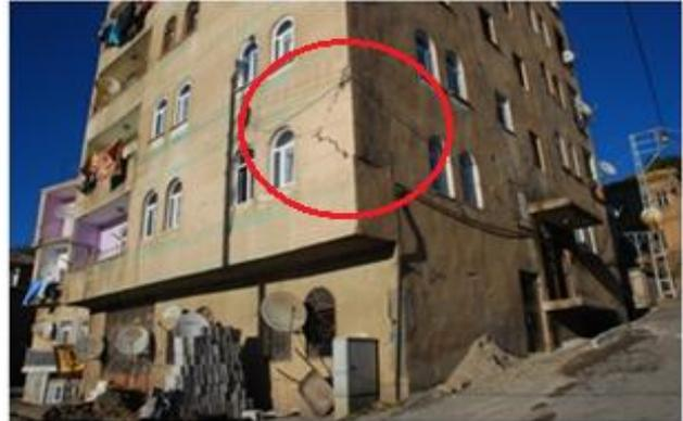
**Fig. 19.** Damages on the large and heavy overhangs
