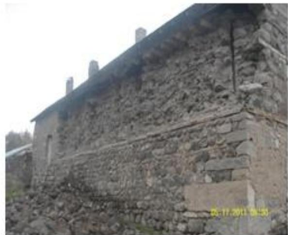
**Fig. 13.** Damages of masonry structures
