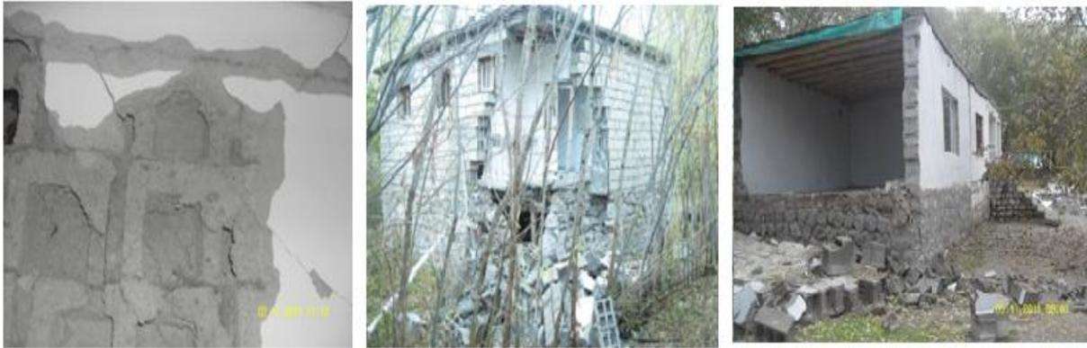
**Fig.9.** Low-strength wall material (briquette) and its damage
