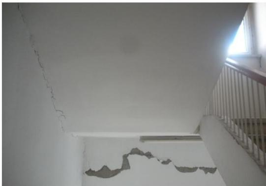
**Fig.20.** Staircase system damage
