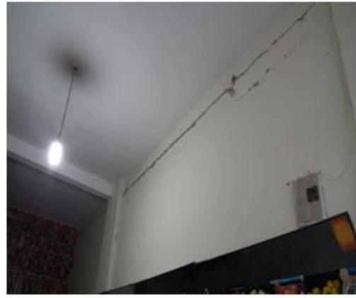
**Fig.12.** Insufficient size of beam and column
