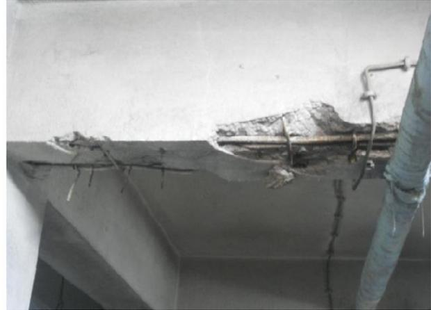
**Fig.24.** Beam damage
