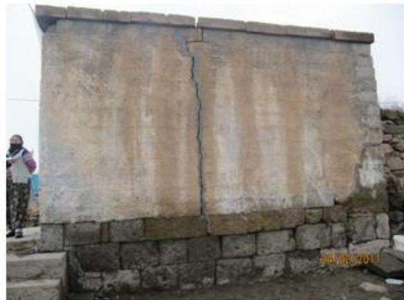
**Fig. 14.** Damages to the poor quality of mortar in Stone structures
