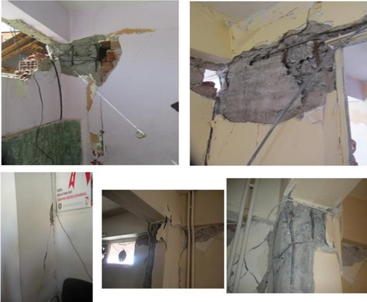
**Fig.26.** Columns damages
