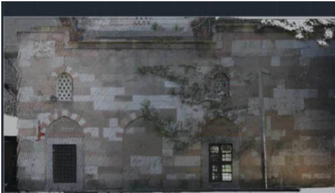
Figure 6. The orthophoto of the west facade produced from TLS data.
